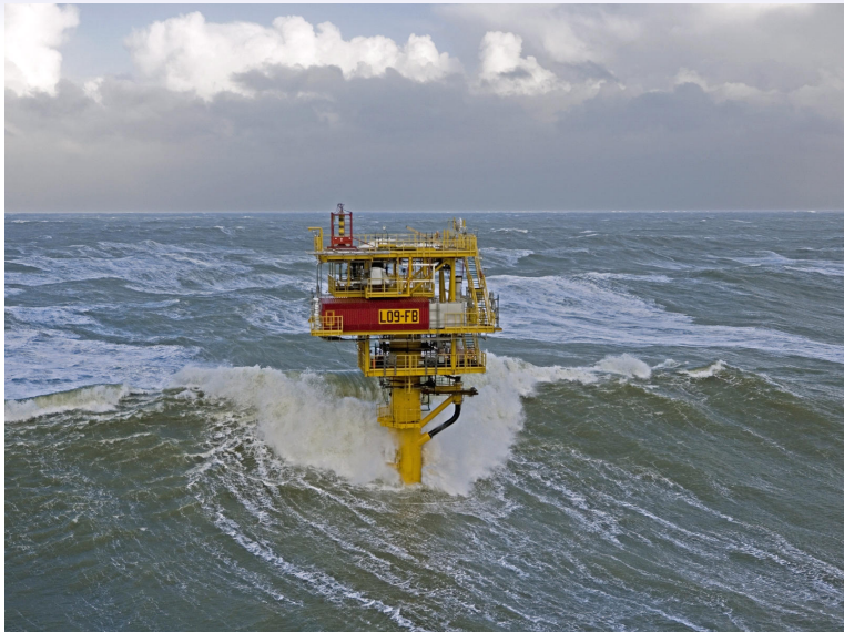
"L9" platform in the Southern North Sea.
